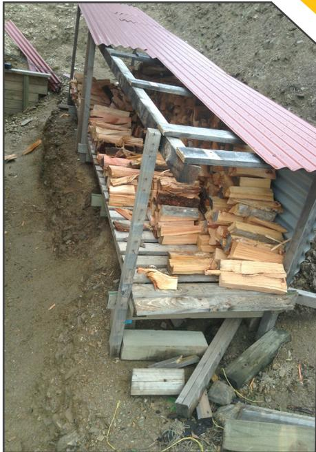
Cut offs from deck posts used to help place pallets on the floor and iron enclosure to create shelter for wood
